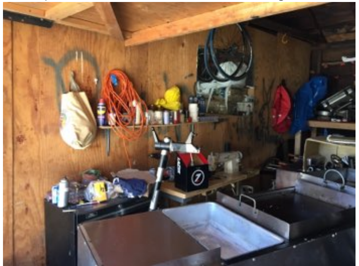
Personal items in garage block complete inspection of all floor, wall and ceiling areas.
