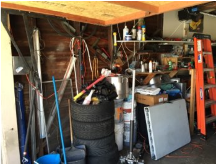
Personal items in garage block complete inspection of all floor, wall and ceiling areas.
