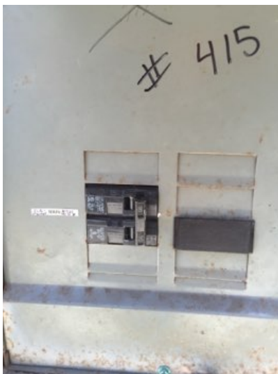
All of the circuit breakers appeared serviceable.
