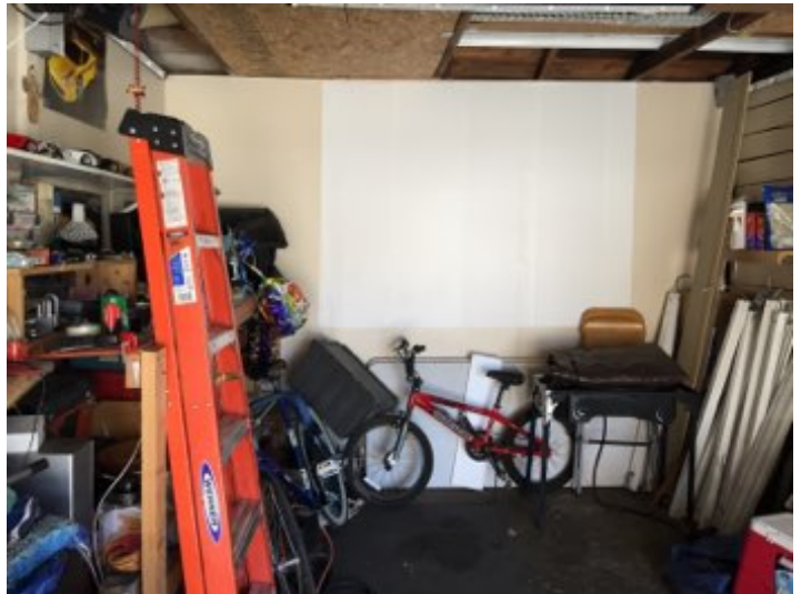
Personal items in garage block complete inspection of all floor, wall and ceiling areas.
