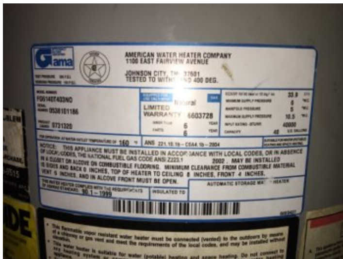
Tank appears to be in satisfactory condition -- no concerns.
