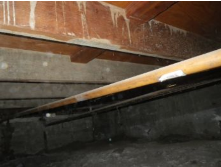
Unsecured supply plumbing observed.
