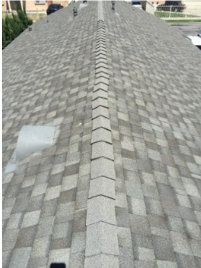
No major system safety or function concerns noted at time of inspection.
