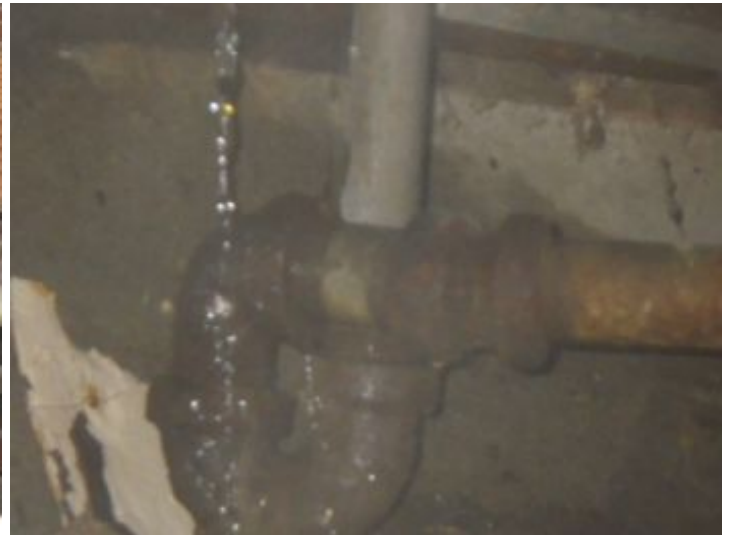
Leaking observed and needs immediate repair by a qualified Plumbing Contractor.
