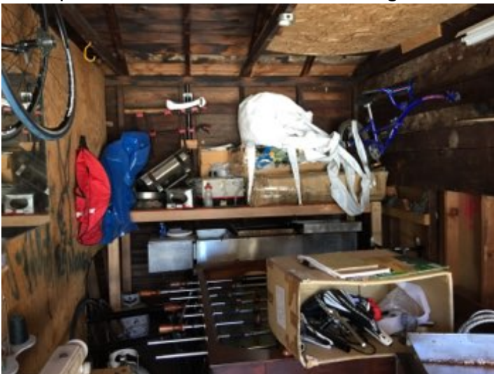
Personal items in garage block complete inspection of all floor, wall and ceiling areas.
