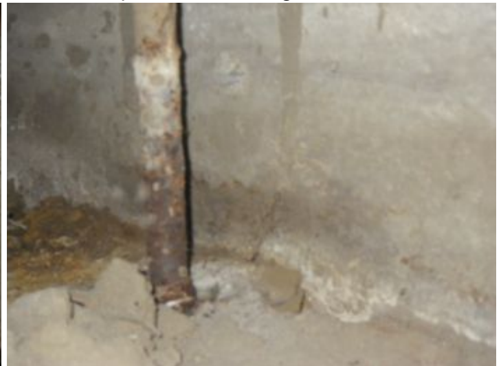
Leaking observed and needs immediate repair by a qualified Plumbing Contractor.
