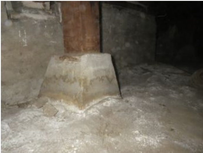
Concrete block/wood piers support floor above.
