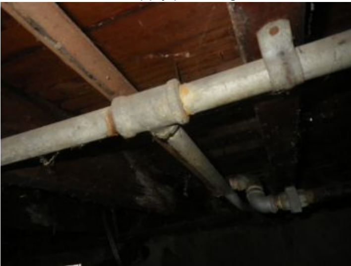
Galvanized pipes present and has an average service life of 30 years. Pipes rust from the inside reducing the diameter and causing loss of pressure and rust in water. Recommend budgeting for replacement of galvanized piping in the near future.
